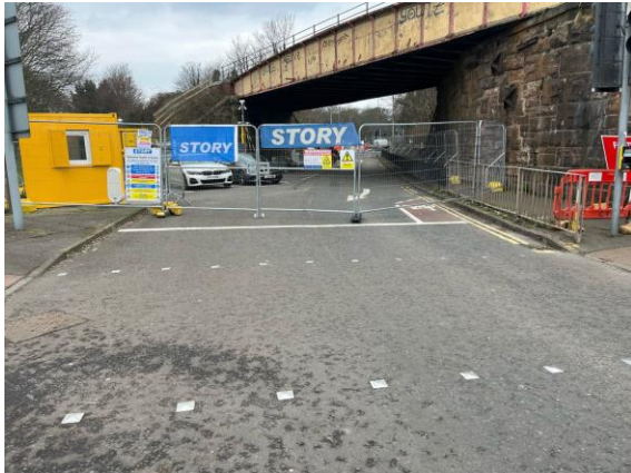
Site compound setup
